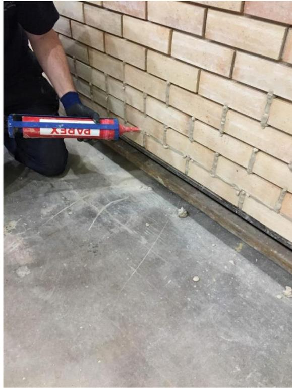
**Plate 7 – Pointing of Brick Slips**
