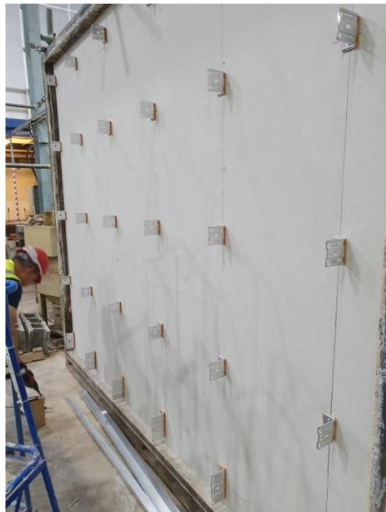
**Plate 2** – Installation of AXL-HB90D-TP Double HB Aluminium Brackets and Pads
