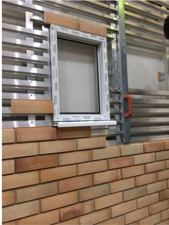
**Plate 5** – Installation of UPC Window
