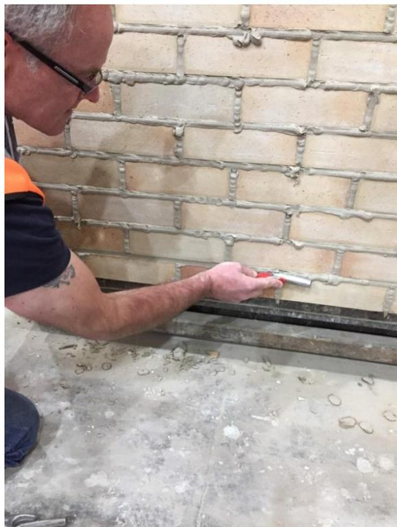
**Plate 8 – Tooling of Mortar**
