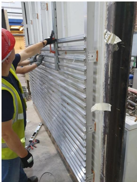
**Plate 4** – Installation of Aluminium Brick Slip Rails
