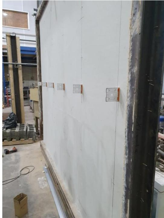
**Plate 1** – Installation of AXL-HB90S-TP Single HB Aluminium Brackets and Pads
