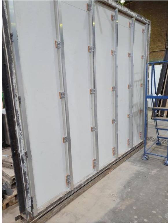
**Plate 3** – Installation of Aluminium Vertical Rails
