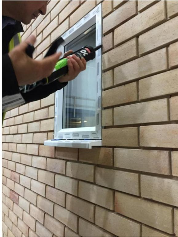
**Plate 9** – Sealing around the Window
